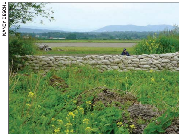
Stillaguamish River, sea dike emergency repair.
