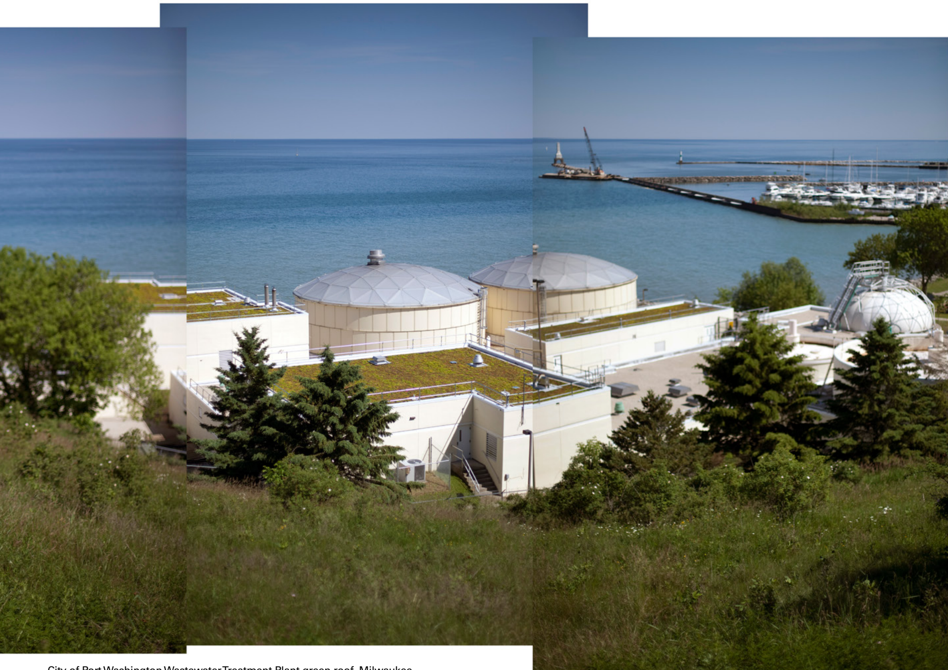
City of Port Washington Wastewater Treatment Plant green roof, Milwaukee
