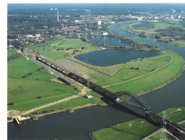
Removal of an hydraulic obstacle, part of the railway bridge at Oosterbeek
