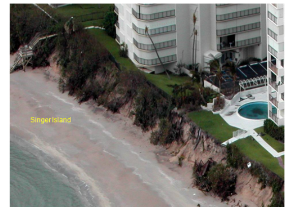
Photo (above): Damage to the Singer Island shoreline in Palm Beach County, Florida after Hurricane Frances. Courtesy of the Department of Environmental Resources Management for Palm Beach County. (October, 2004).
