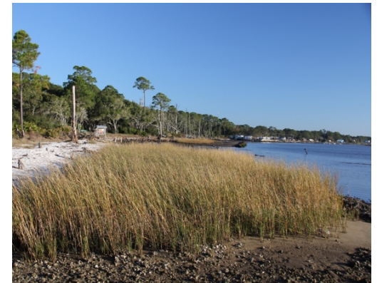
Photo (right): A living shoreline restoration project (an example of soft armoring) in Millender Park in Eastpoint, Florida. Photo courtesy of the Apalachicola National Estuarine Research Reserve (2015).
