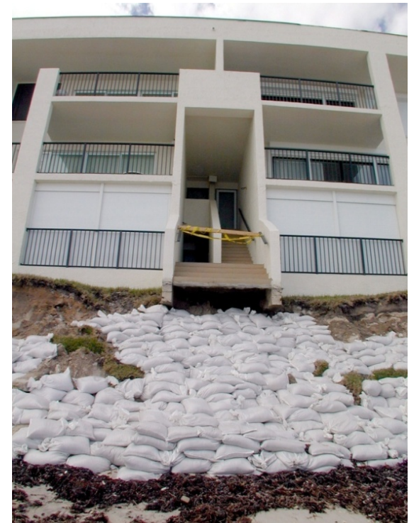
Photo (above): Melbourne Beach, FL, The Breakers Resort is at continued risk following beach erosion caused by Hurricane Irene. The Federal Emergency Management Agency's (FEMA) PROJECT IMPACT is working to assist communities with steps they can take to make residents and property safer and more disaster resistant. Photo by Ty Harrington/FEMA News Photo (October 1999)
