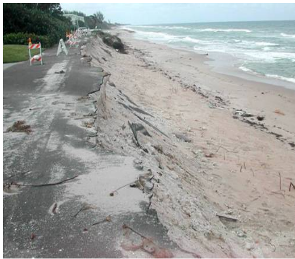
Photos (above): Road erosion on Old South Ocean Boulevard due to Hurricane Frances in 2004 in Palm Beach County, Florida (before and after). Courtesy of the Palm Beach County Department of Environmental Resources Management (2004).
