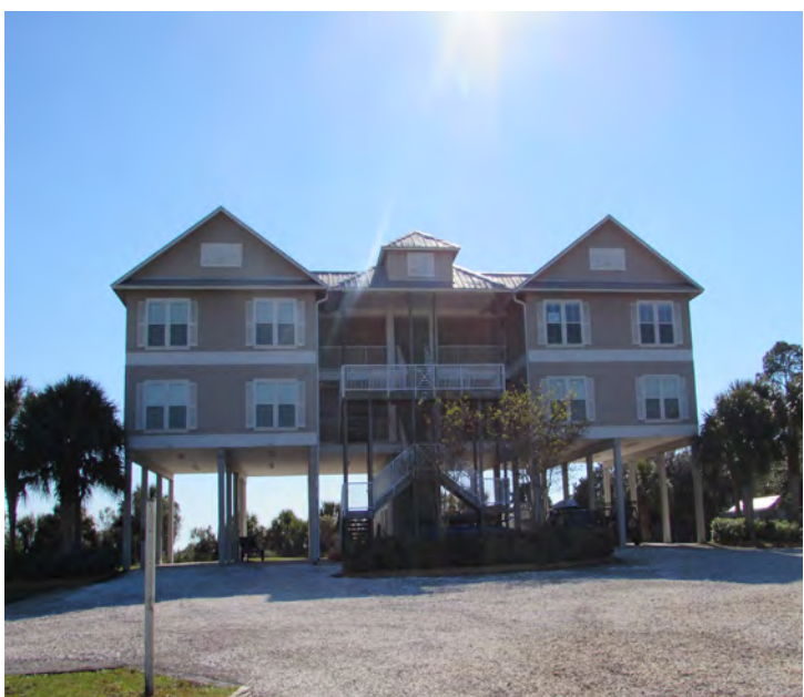
Elevated coastal structure
