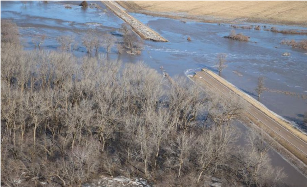
Figure 15. Highway 39 Bridge South of Genoa, Nebraska (State of Nebraska)
