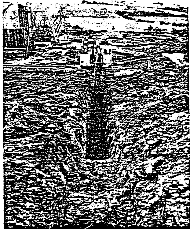
Fig. 10: Photograph of trench drain being dug in a till slope at Low Worsall, Yorkshire, April - May 1977 (with acknowledgements to the Northumbrian Water Authority).
