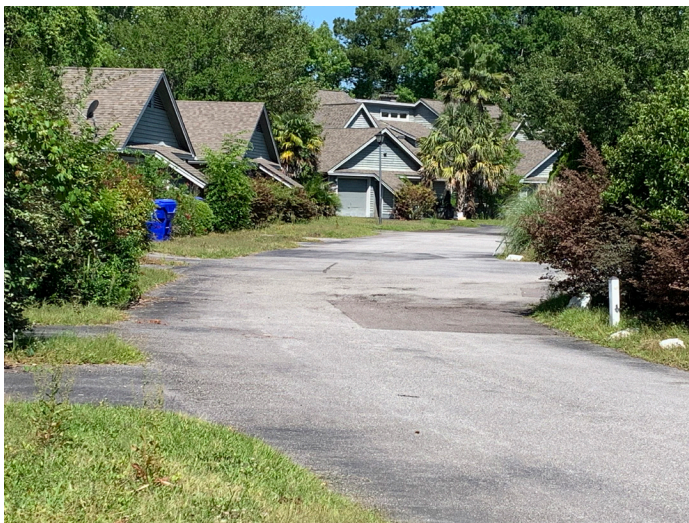
Repeatedly flooded townhomes await demolition in the West Ashley area of Charleston, SC.
