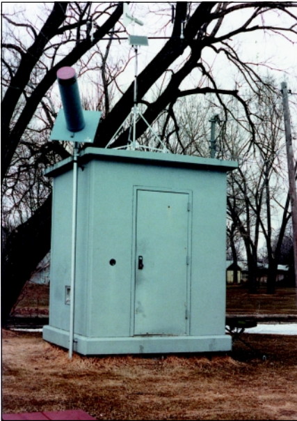
Typical water level gaging station with satellite data relay instrumentation
