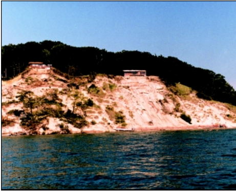
High bluff along Lake Michigan shoreline
