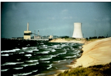
Power plant and dunes on Lake Michigan shoreline in Indiana
