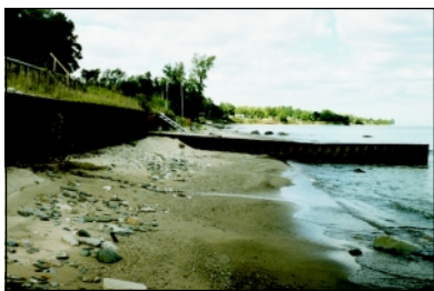
A bulkhead and companion breakwater in Sanilac County, Michigan, on Lake Huron
