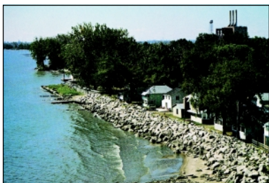
Revetment at Luna Pier, Michigan, on Lake Erie
