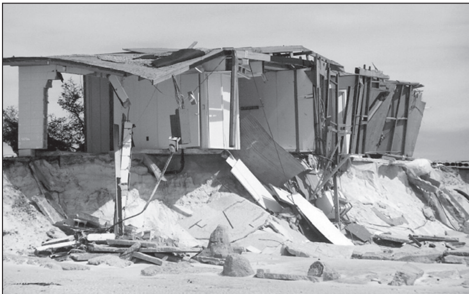
Figure 3-8. Large, fast-moving waves combined with erosion and scour to destroy this Gulf of Mexico home during Hurricane Opal
