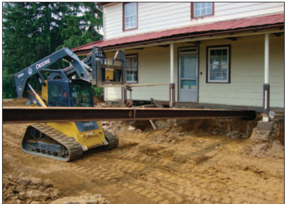
Figure 5R-6. Beams supported by cribbing are placed at critical lift points (photo courtesy of Wolfe House Movers)
