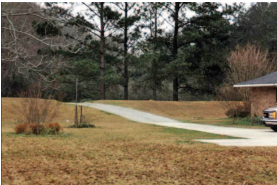
Figure 6-57. Driveway access over a residential levee
