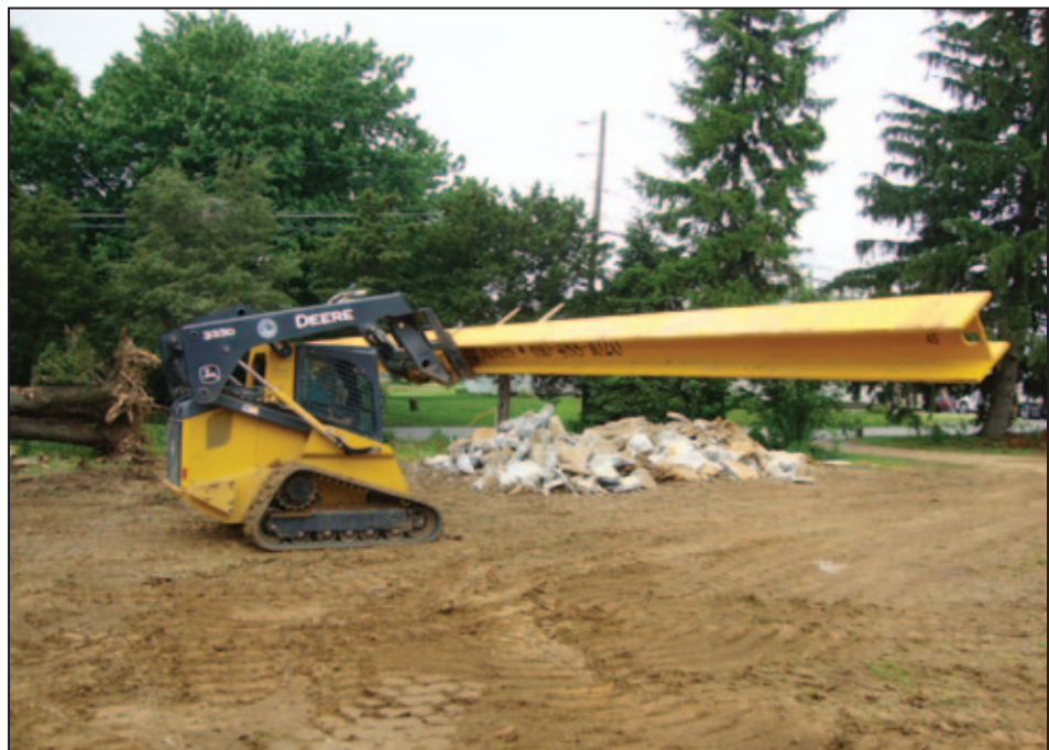
Figure 5R-9. Foundation preparation at new site (photo courtesy of Wolfe House Movers)
