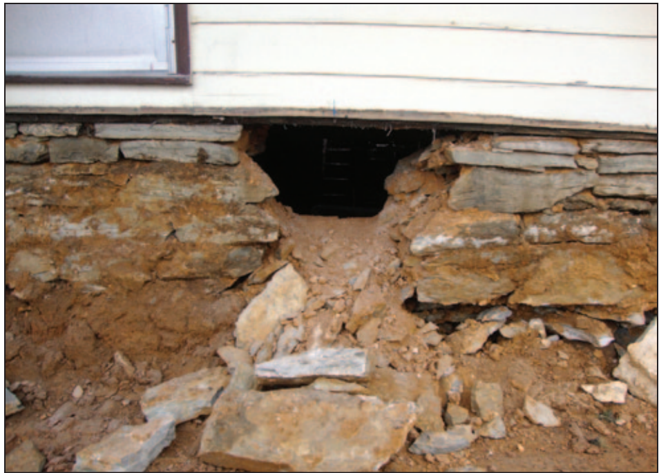
Figure 5R-4. Clearing pathways beneath the structure for lifting supports (photo courtesy of Wolfe House Movers)
