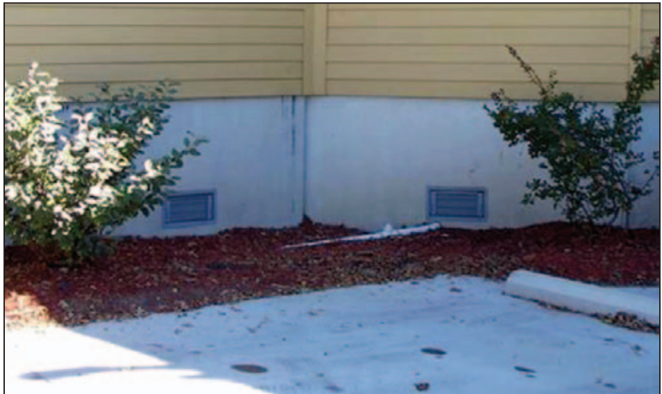
Figure 6-42. Example of flood vents
