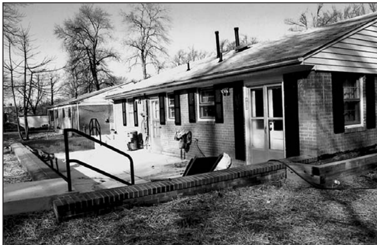
Figure 6-55. Brick-faced residential floodwall and access stairs
