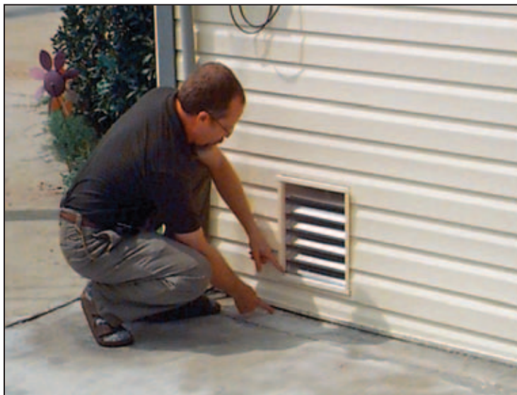
Figure 6-43. Example of flood vents
