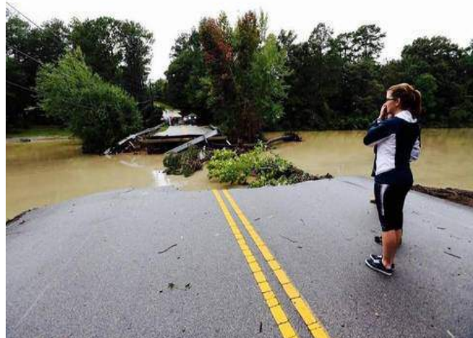
A resident of a nearby home looks at the destruction caused by the Arcadia Lakes dam failure (Source: Matt Walsh)
