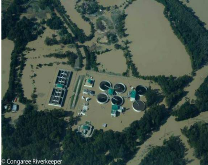
A water treatment facility in Columbia, SC is engulfed in floodwater. (Source: Congaree Riverkeeper via WIS-TV)
