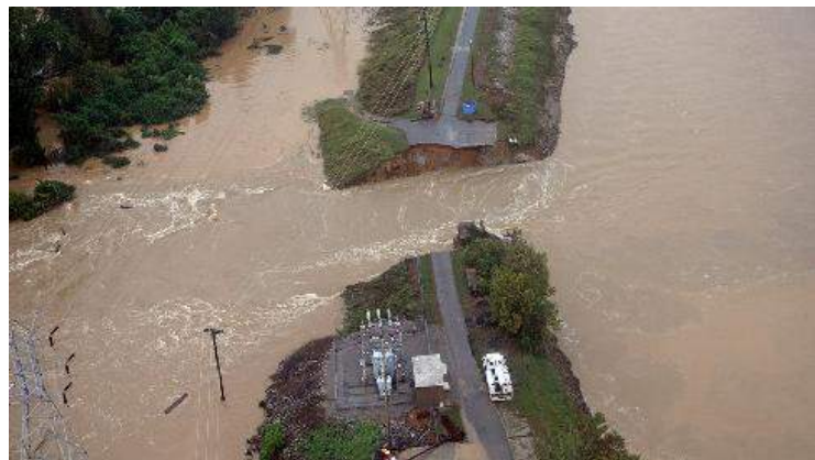
Floodwaters destroyed many roadways by eroding the land underneath (Source: AP/Chuck Burton via Weather.com)
