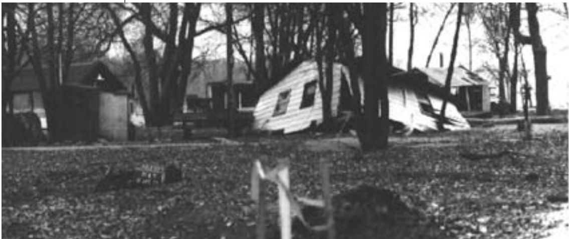
Substantially damaged home in Calhoun County, Illinois bought out after 1993 flood. Photo: Illinois Department of Natural Resources
