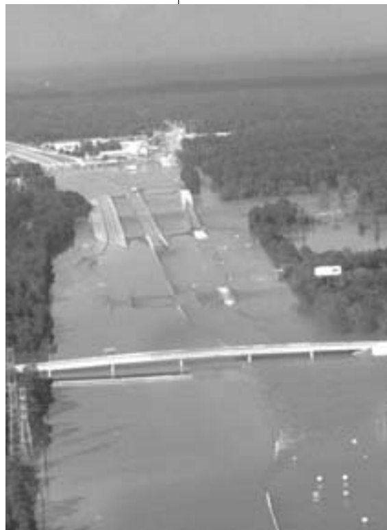
The Interstate east of Houston was closed when only the overpasses were above water. Photo: U.S. Army Corps of Engineers
