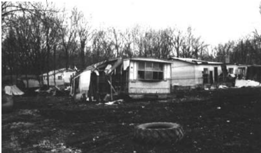
Flood damaged mobile homes in E. Harden, Illinois in October 1993. Since that time the homes were bought out. Photo: Illinois Department of Natural Resources
