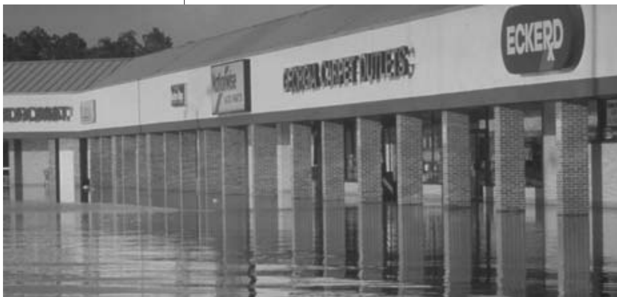
Strip mall closed in Albany, Georgia after floodwaters reach waist high. Photo: U.S. Army Corps of Engineers
