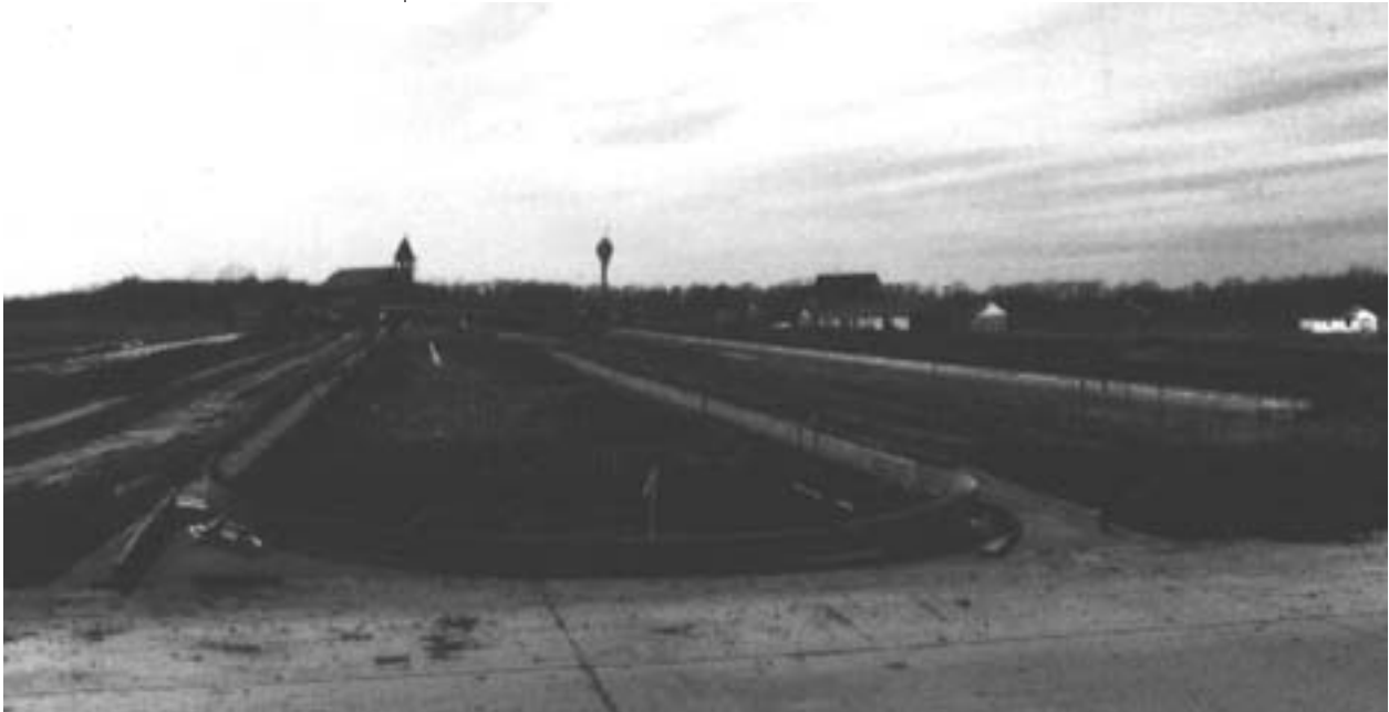
New Valmeyer, Illinois under construction. After the 1993 Midwest Flood, residents of Valmeyer decided to move their town off the Mississippi bottoms to higher ground. Photo: Illinois Department of Natural Resources
