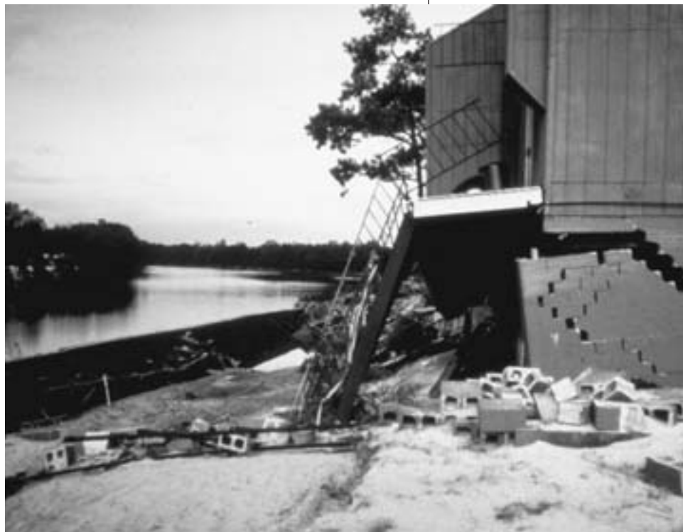
Flooding wreaks havoc for a homeowner along a river in Texas. Photo: FEMA
