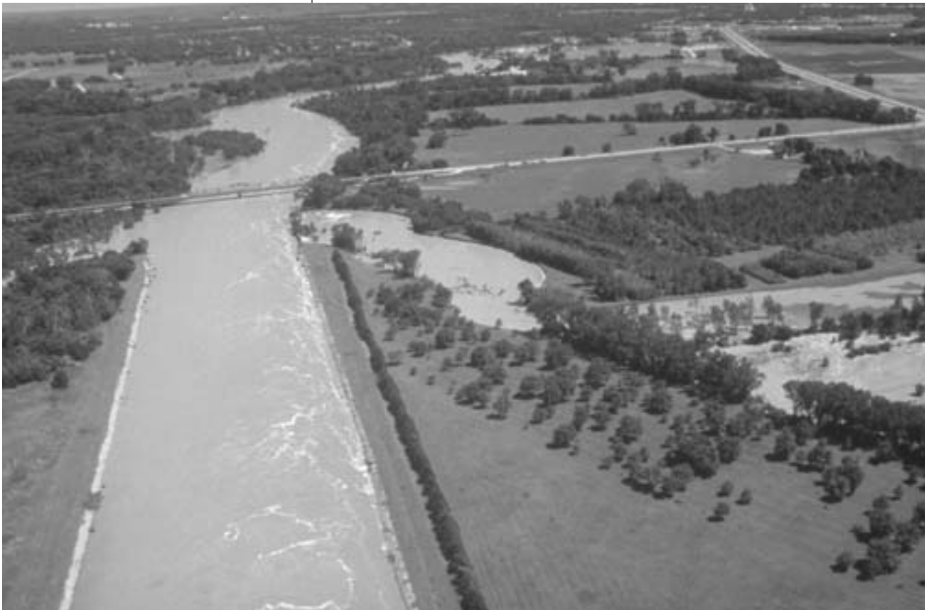
River channelled by levees in Republican, KS, July 25, 1993. Photo: National Oceanic and Atmospheric Administration
