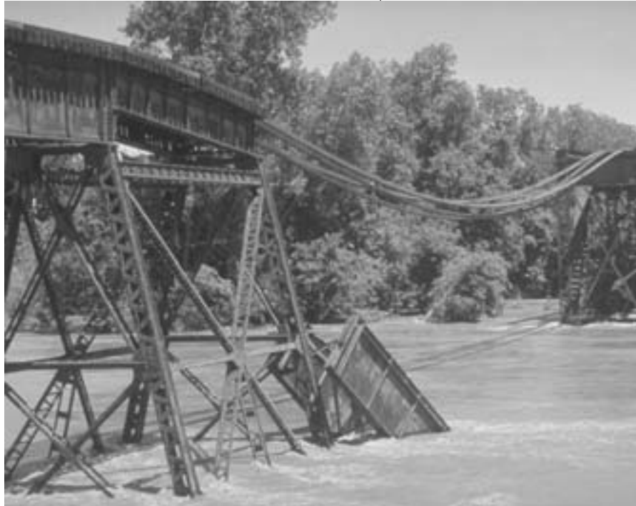
Glasgow, Missouri railroad bridge destroyed in flooding. Photo: NOAA
