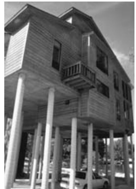
In fall, 1994, some houses were built on stilts to avoid flooding in Galveston, Texas. Photo: FEMA
